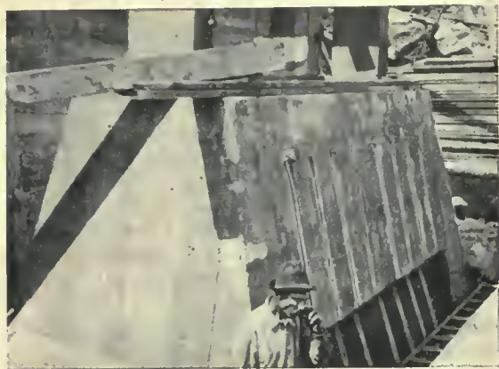
STAMP FOUNDATIONS AT BISHOP CREEK MILL.
